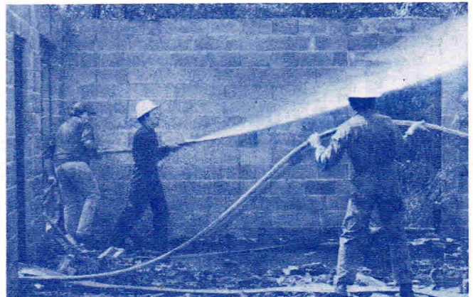
An old house site in bush at Padthaway was used to demonstrate the need for assistance to the lead fireman in carrying hoses around corners. photos courtesy 'Border Chronicle'.
